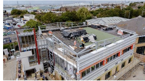
Figure 13: Installation of the Biosolar roof at East Kent College
